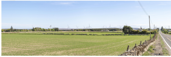
Looking towards Loch Toftingall BESS site with Halsary Wind Farm in the background
