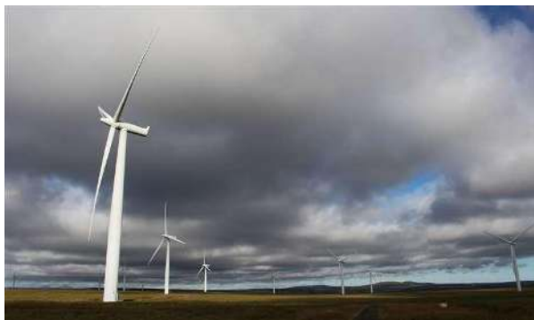
The Causewaymire is already home to a number of wind turbines. Picture: Alan Hendry
